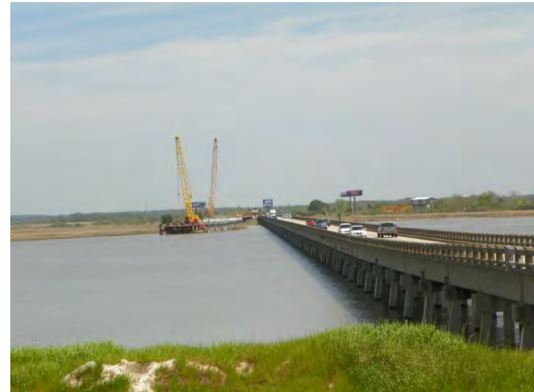
Photograph 4. Previous bridge over the Back River and location of the proposed bridge.
